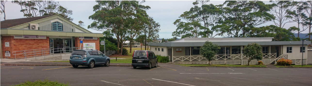
The Te Atatu South Community Hall and the St John Hall at Lloyd Morgan Park in Edmonton Road
