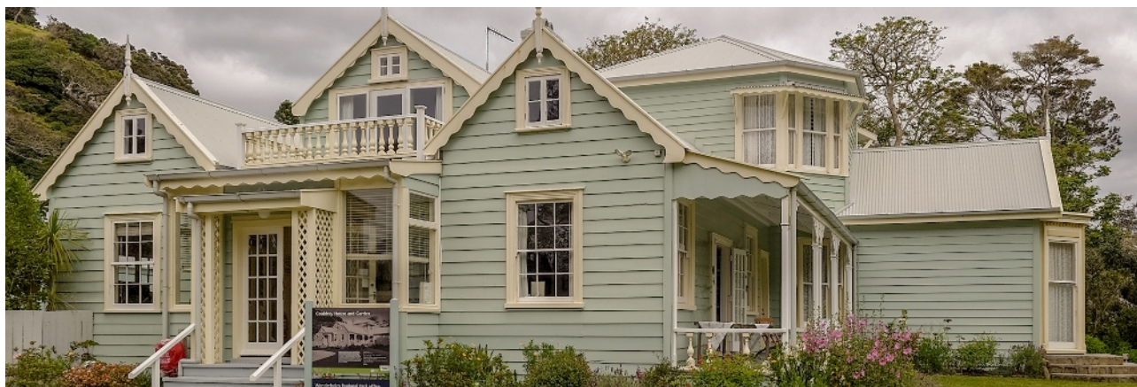
Couldrey House is an historic Victorian-Edwardian family home in Wenderholm Regional Park
