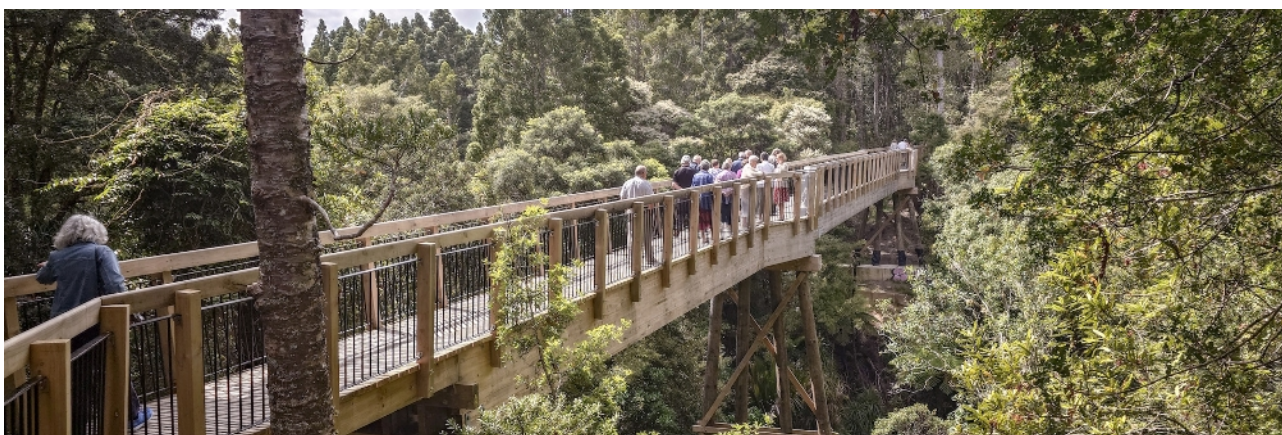
The Kauri Glen tree top boardwalk is 60 metres long and 18 metres high
