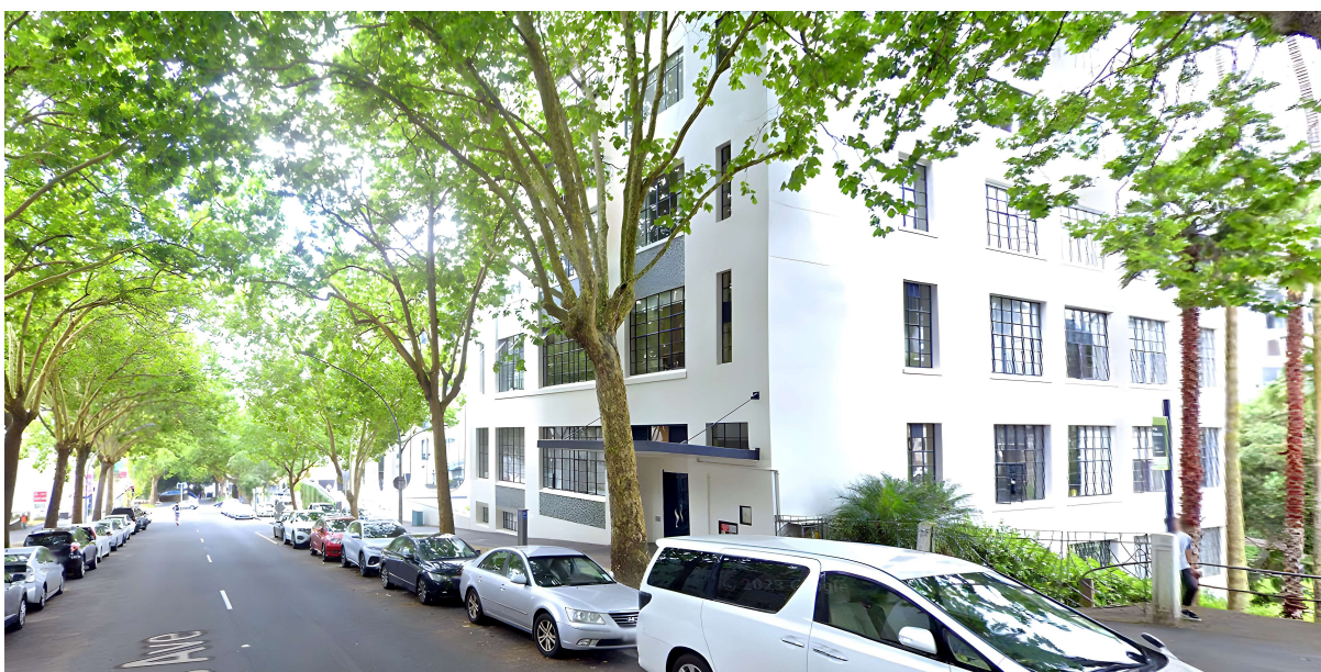
Waitemata City Council building in Grey's Avenue
