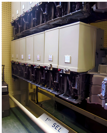
Telephone exchange selectors
