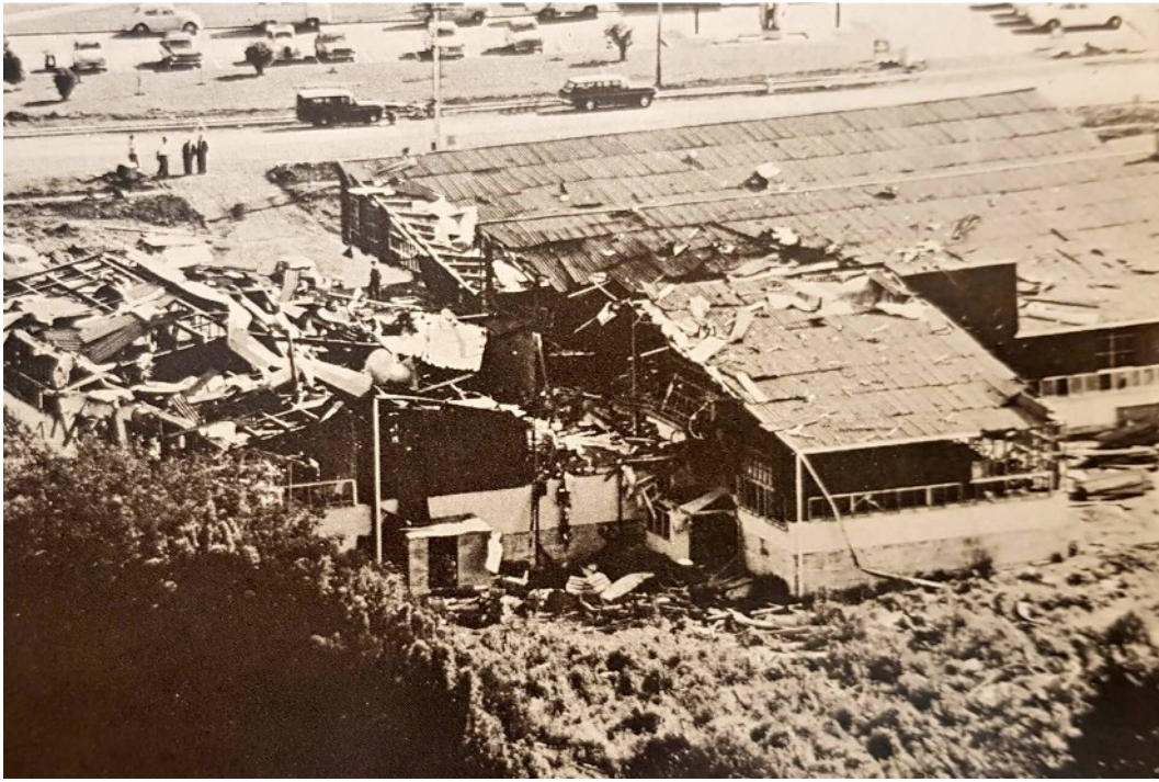
The explosion wrecked the F.&W. Fowler building and blew out every window within half a mile radius
