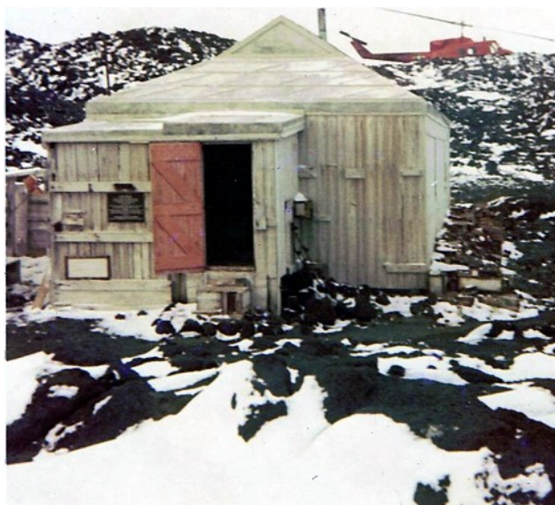
Shackleton's Hut erected at Cape Royds in early 1908
