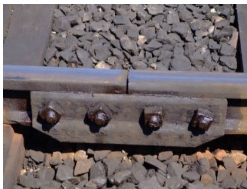
A fishplate is a metal connecting plate used to bolt the ends of two rails into a continuous track
